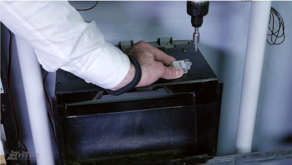
**8. Connect the receiver wire harness to the CPU.**
